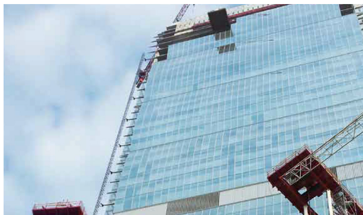
The Allianz Tower in Milan, Italy is a 50-story skyscraper that was constructed with 80,000 cubic meters of concrete using Buzzi Unicem's PLC Type II/A-LL.
